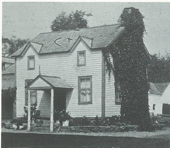
Watson house after rebuilding.
