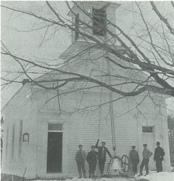
Installing new bell at church
