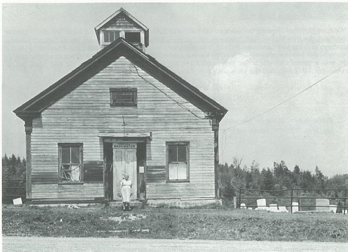
Picture as it looked before work started.
