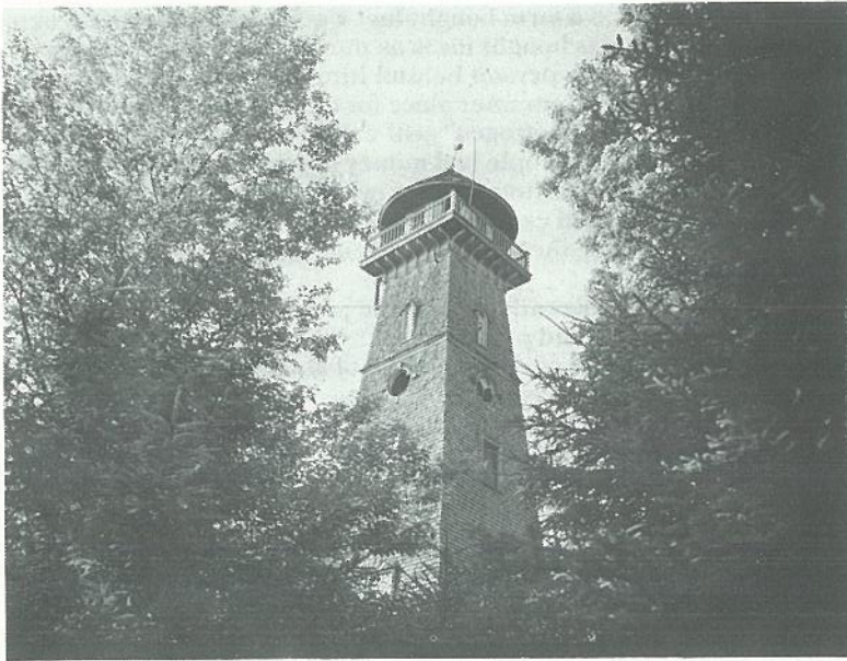
Tower on Whitney Estate.
